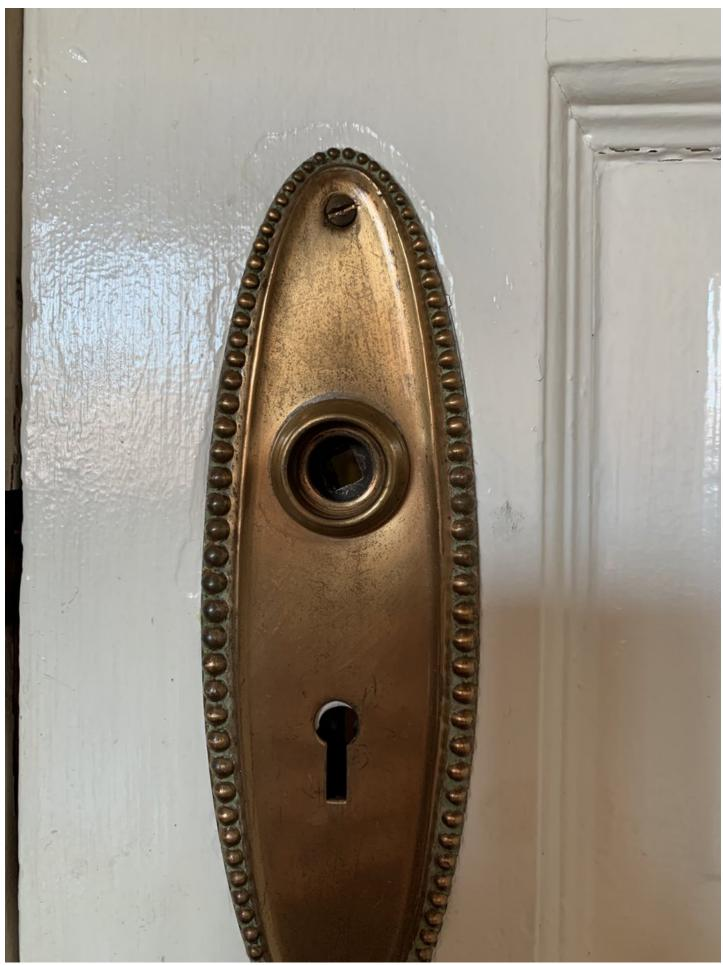
Those suggesting I just disassemble the latch, it is fully inside the door (which is over 100 years old and original to the house). That square hole still turns. It just isn't connected to whatever opens the latch.
