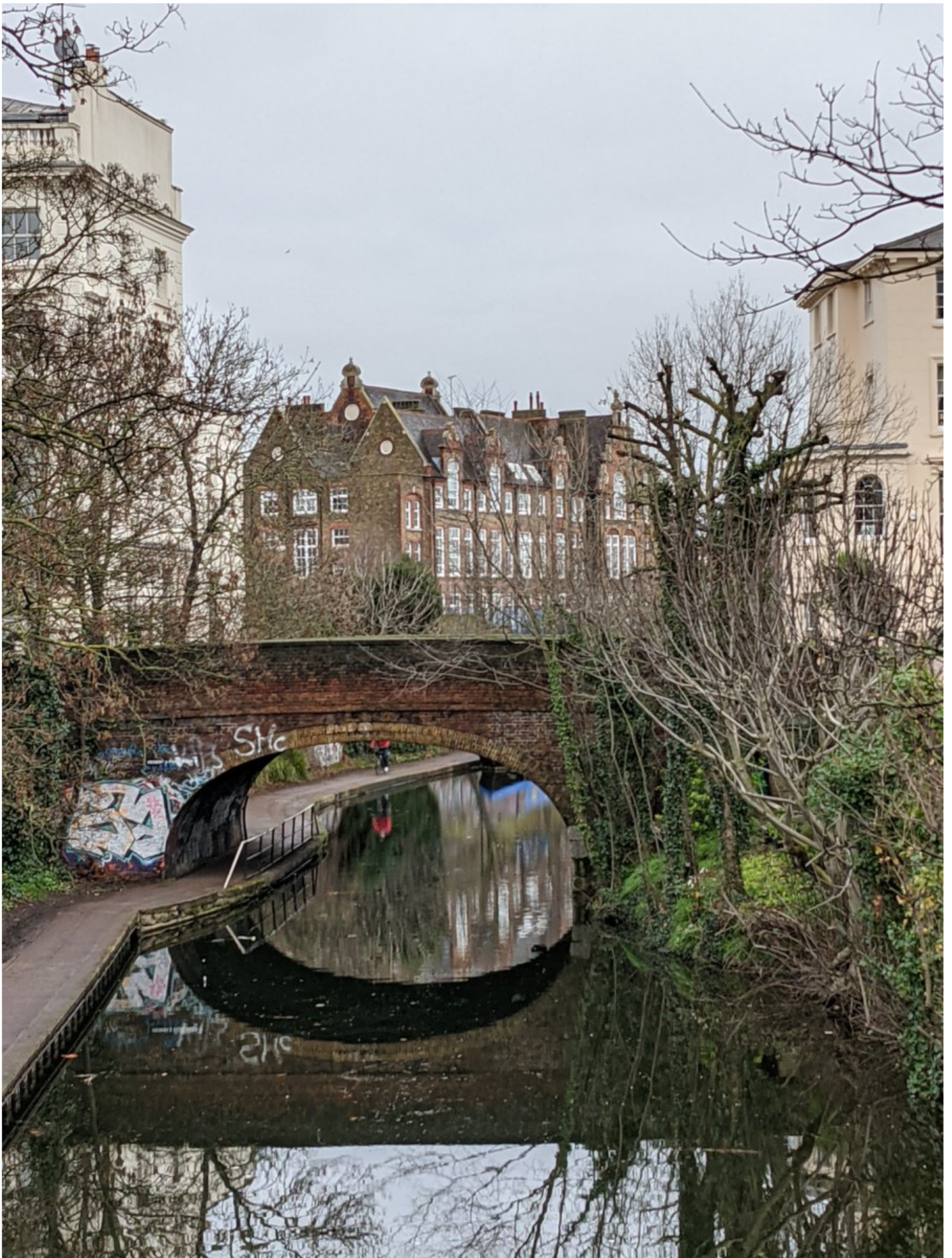
6/ Water Meeting Bridge, over the Regent's Canal, rebuilt by St Pancras Metropolitan Borough Council in 1961. Borough Motto: 'With Wisdom and Courage'.
