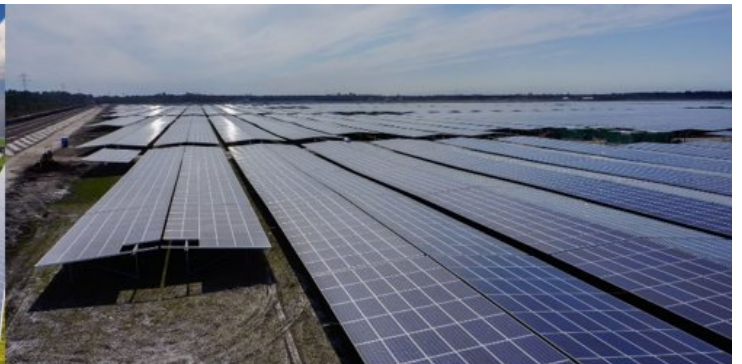
East-west configuration: cover over 80%
